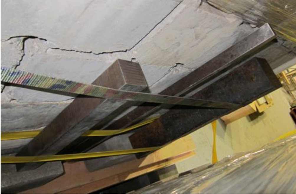
Figure 5: The iron bars inside the wall. Image by authors.
