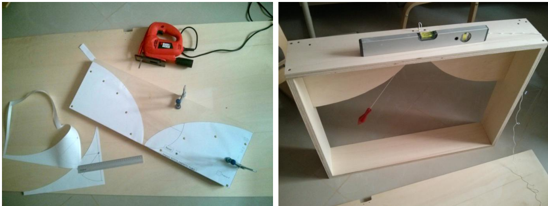
Fig. 7. Two steps in the realisation of the Heygens' pendulum: the use of printed cycloid from Geogebra (on the left side) and the levelling of the device (on the right side).
